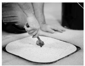
Using a trowel or roller, embed the cover membrane into the cold process adhesive (mastic) completely and evenly while leaving a ¼ **inch bleed out** around the perimeter of the cover membrane.
